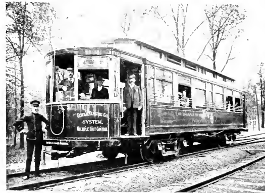
FIG. 4.—A CAR ON THE ELECTRIC RAILWAY.
